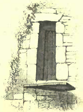
DOORWAY OF ROUND TOWER, CLONDALKIN.
